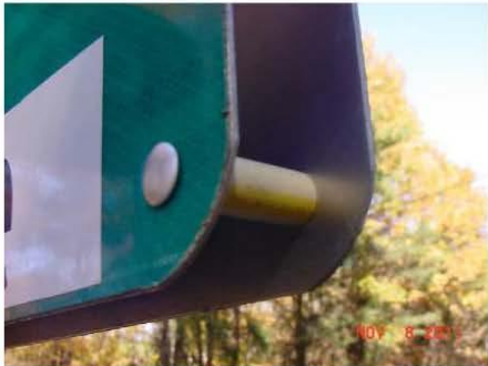
Figure III-7 Oversize Sign Showing 2'' Spacer (Gab) Detail
