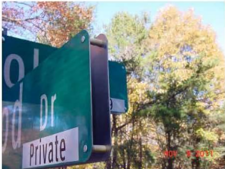
Figure III-8 Oversize Sign Showing Corner Attachment Detail
