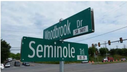
Figure III-6 Oversize (12'') Sign Showing Direct Mount Method
