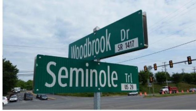
Figure III-6 Oversize (12'') Sign Showing Direct Mount Method
