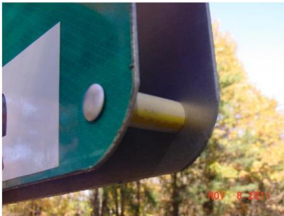
Figure III-7 Oversize Sign Showing 2'' Spacer (Gab) Detail
