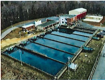
South & North Fork Rivanna Water System
