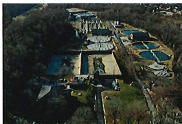
Moores Creek Advanced Water Resource Recovery Facility (Wastewater)
