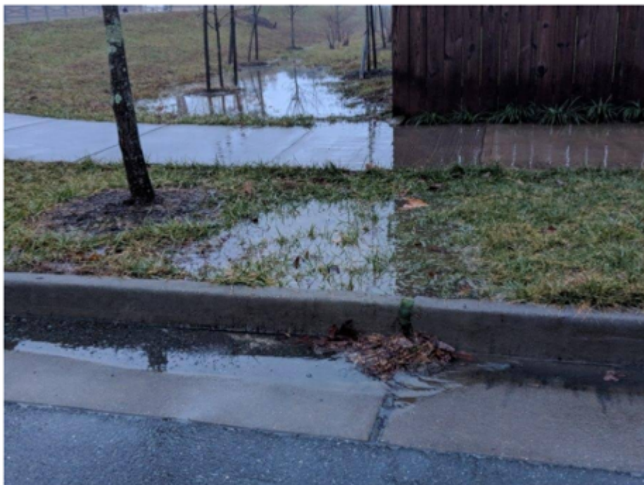
Figure 3 – Water flowing over sidewalk, which can create a slip hazard during freezing weather.
