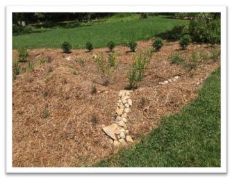
This home had two downspouts draining to a steep slope close to a stream. With ACAP, two small rain gardens were installed to capture runoff from the house and the lawn. The homeowner installed these practices to increase the infiltration of runoff and help prevent erosion of the hill and stream bank downslope.
