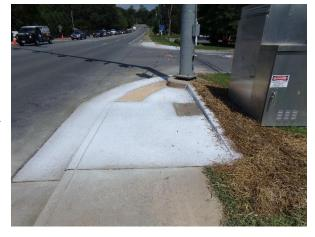
Construction started in June of 2020, adding underground conduit and wiring to the feed new pedestrian crossing notification signal
