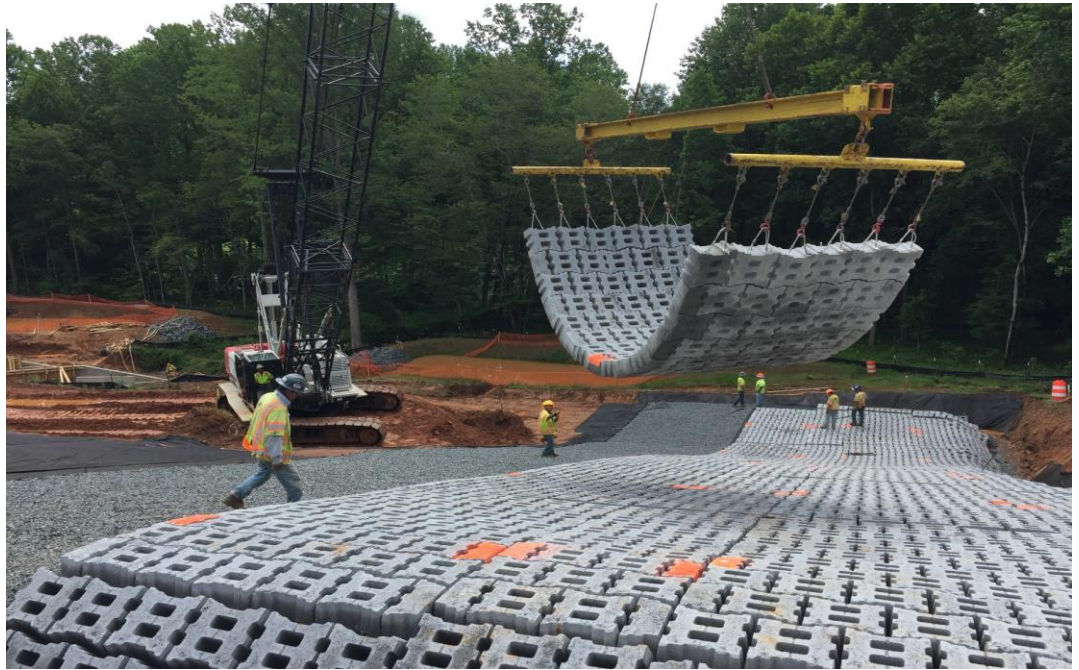
Installation of articulated concrete blocks
