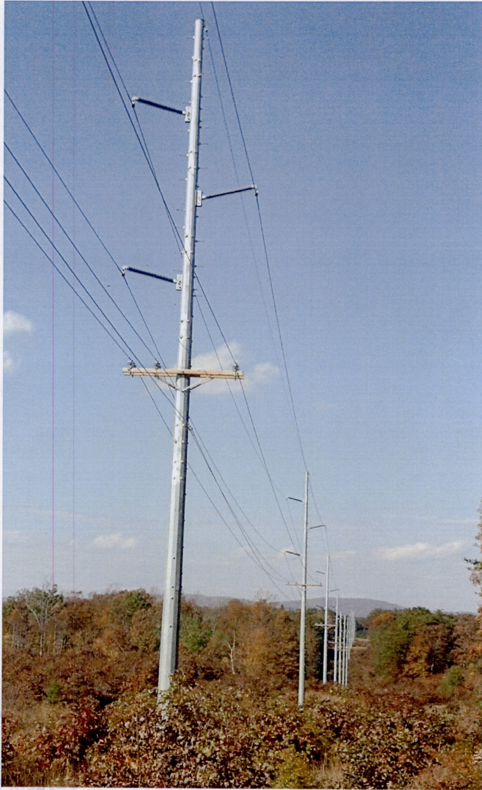
NEW 115 KV LINE WITH 25 KV DISTRIBUTION UNDERBUILD POLES WILL BE BROWN WEATHERING STEEL NOT GALVANIZED STEEL AS SHOWN
