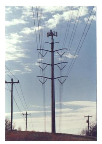
Pictured is an antenna array on top of a transmission tower along Barracks Road. While this represents use of an opportunity site, the resulting design has visibility impacts that could have been reduced or eliminated by using alternative types of equipment and mounting techniques. Attachment to existing structures should complement - not overwhelm - the structure
