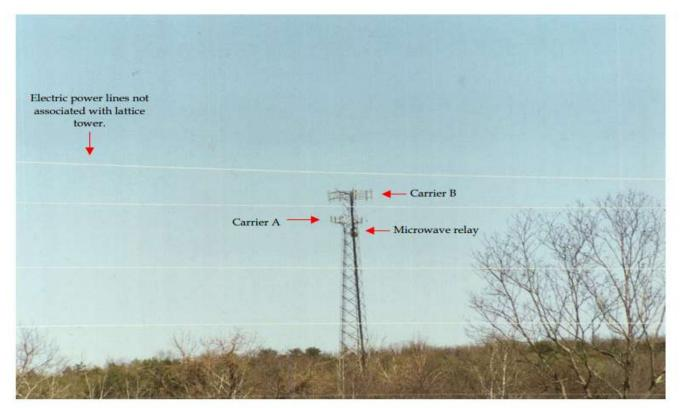
This is a tri-location of personal wireless service facilities near Boyd Tavern on a lattice tower. The microwave relay can be used for backhaul by both Cellular and PCS carriers, which also use wireline (telephone) for backhaul when it is readily available.
