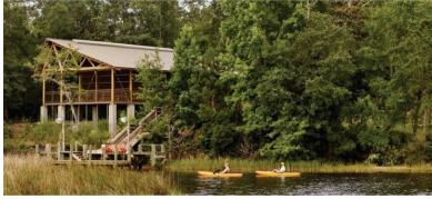
By supporting a structured floor on point loded pier footings we are able to avoid grading large portions of the site. The result is that the building will appear to hover just above the ground and the natural landscape will be allowed to exist undisturbed.
