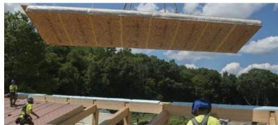
By utilizing *a prefabricated panel system* we are already prepared for disassembly when the time comes for the buildings to be deconstructed...
