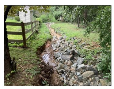
deteriorated to the point of causing impacts on multiple properties. One such case in the Mill Creek neighborhood is pictured above. A particularly intense storm displaced riprap and caused eroded, incised, and unstable area. If not addressed in a comprehensive manner, inadequate channels would likely worsen over time and, perhaps, increase the risk of property damage due to extensive erosion or flood.
