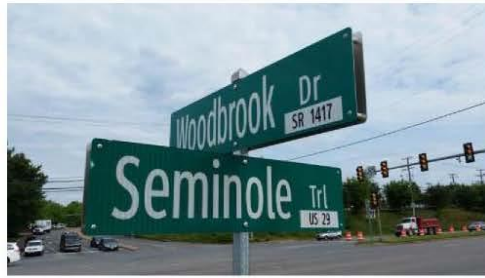
Figure III-6 Oversize (12'') Sign Showing Direct Mount Method
