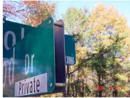
Figure III-8 Oversize Sign Showing Corner Attachment Detail
