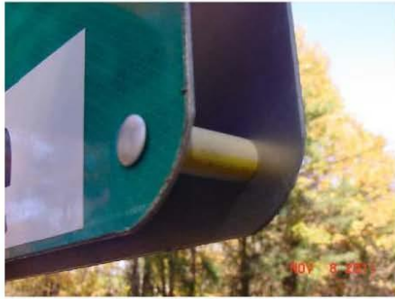
Figure III-7 Oversize Sign Showing 2'' Spacer (Gab) Detail
