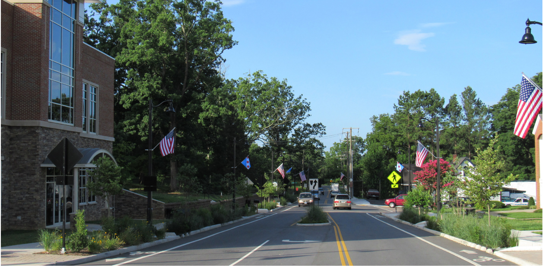
Crozet Avenue, Downtown Crozet (Crozet Library on the left). Example of a complete street, with bicycle lanes, sidewalks, and greenery on both sides.
