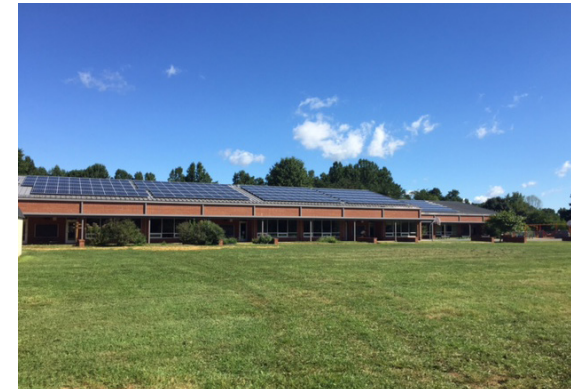
Rooftop solar installation at Brownsville Elementary School in Albemarle County.
