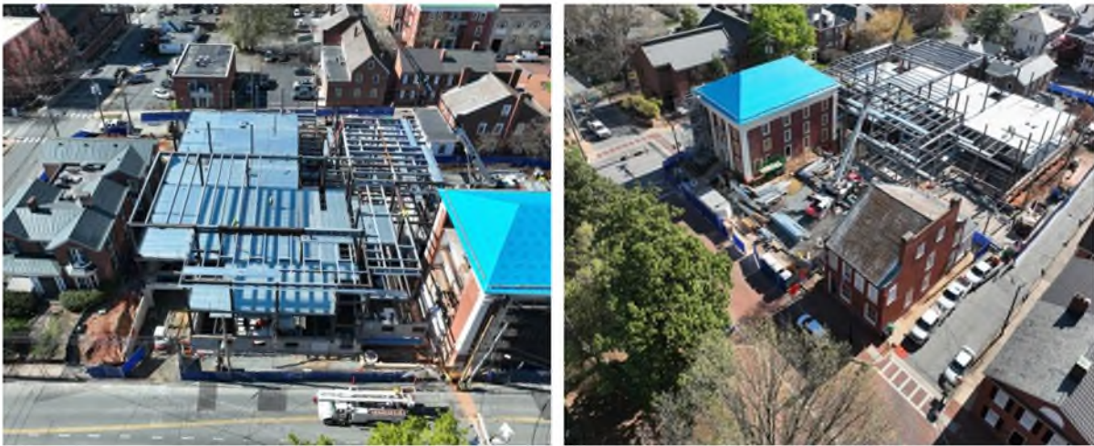
Steel and decking being installed.
