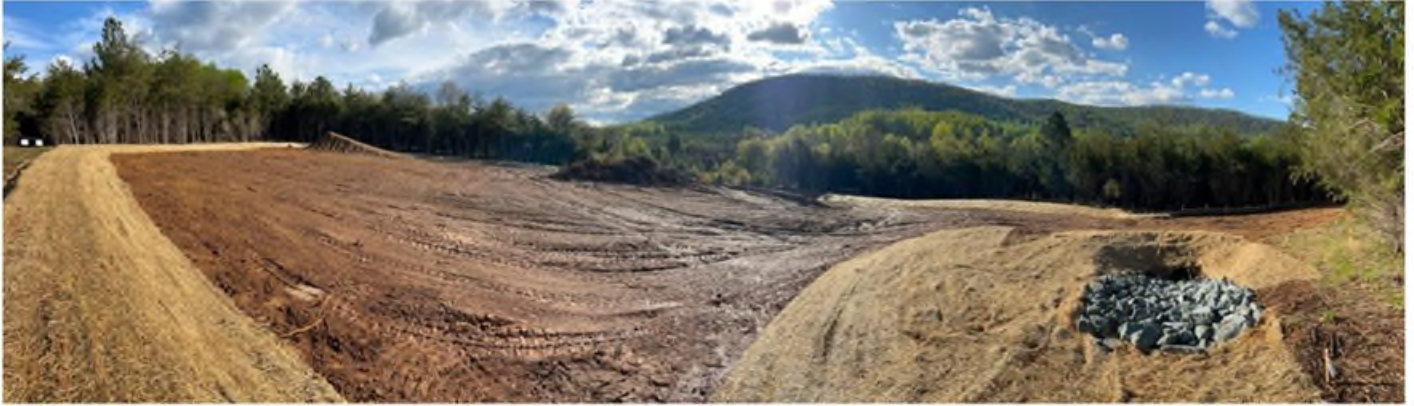
Grading and erosion control.
