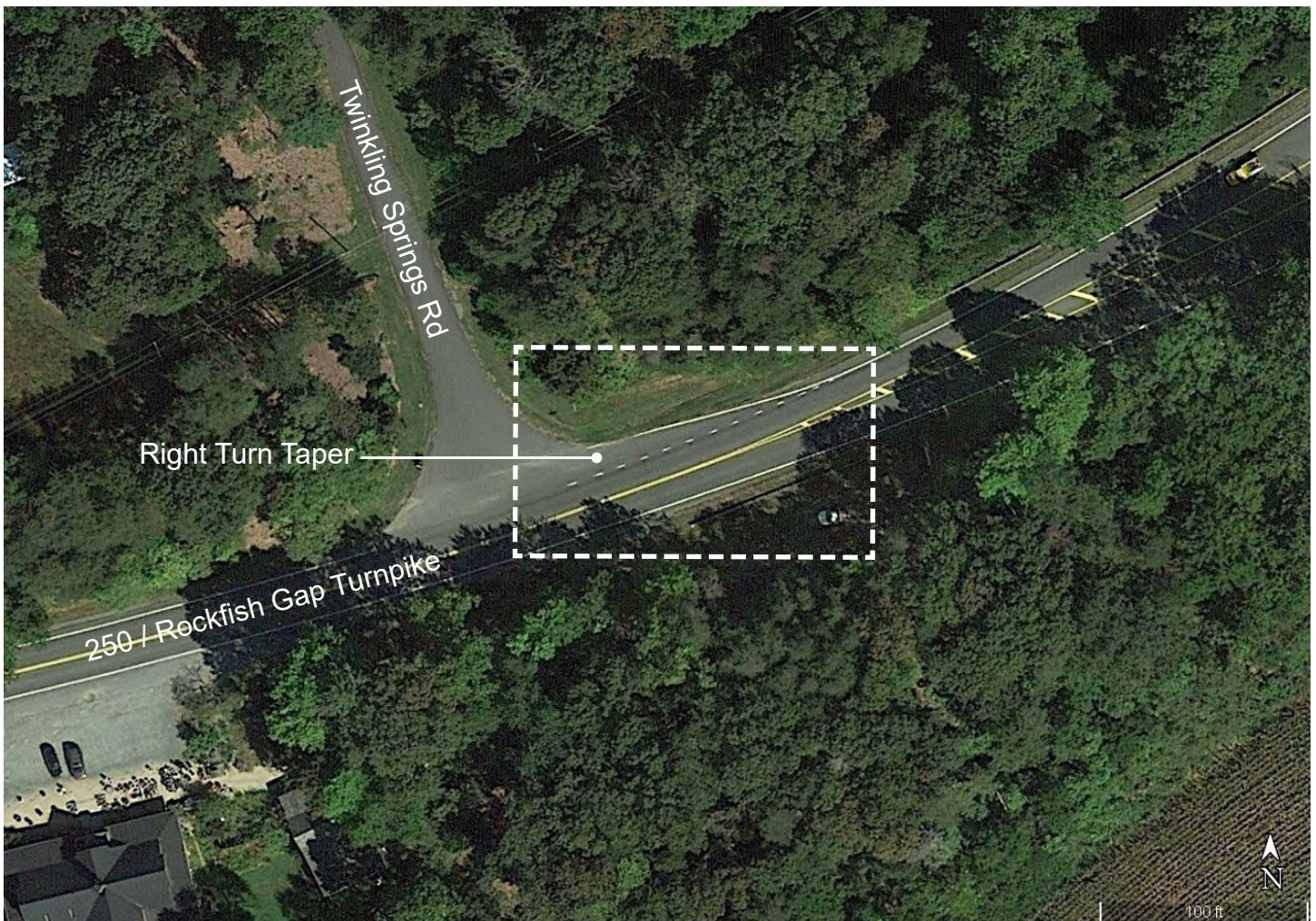
Figure 4 – Existing Right Turn Lane
