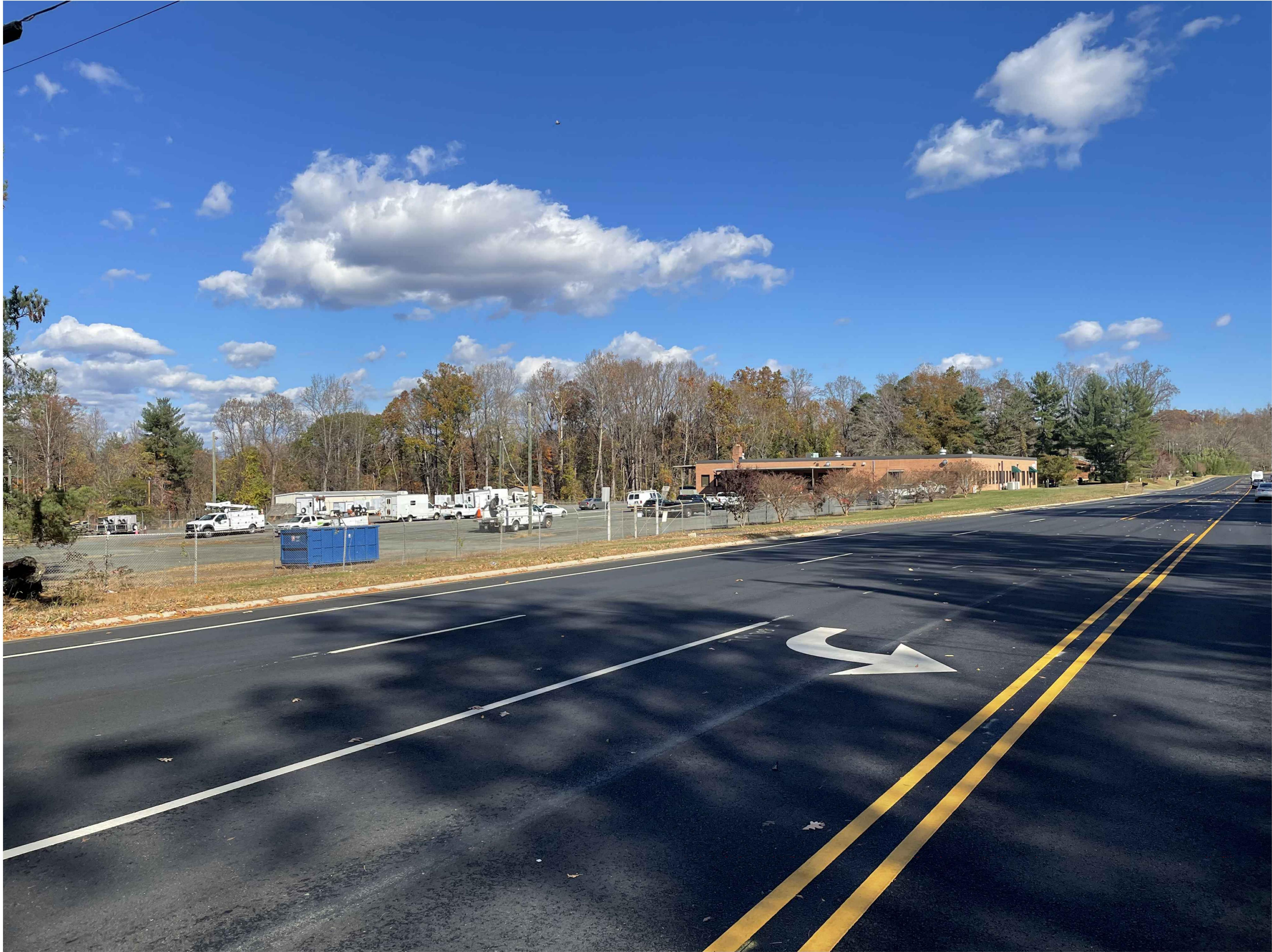
EXISTING FRONTAGE CONDITION - WEST ENTRANCE VIEW
