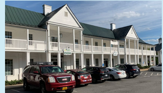
Existing commercial use building, North Garden
