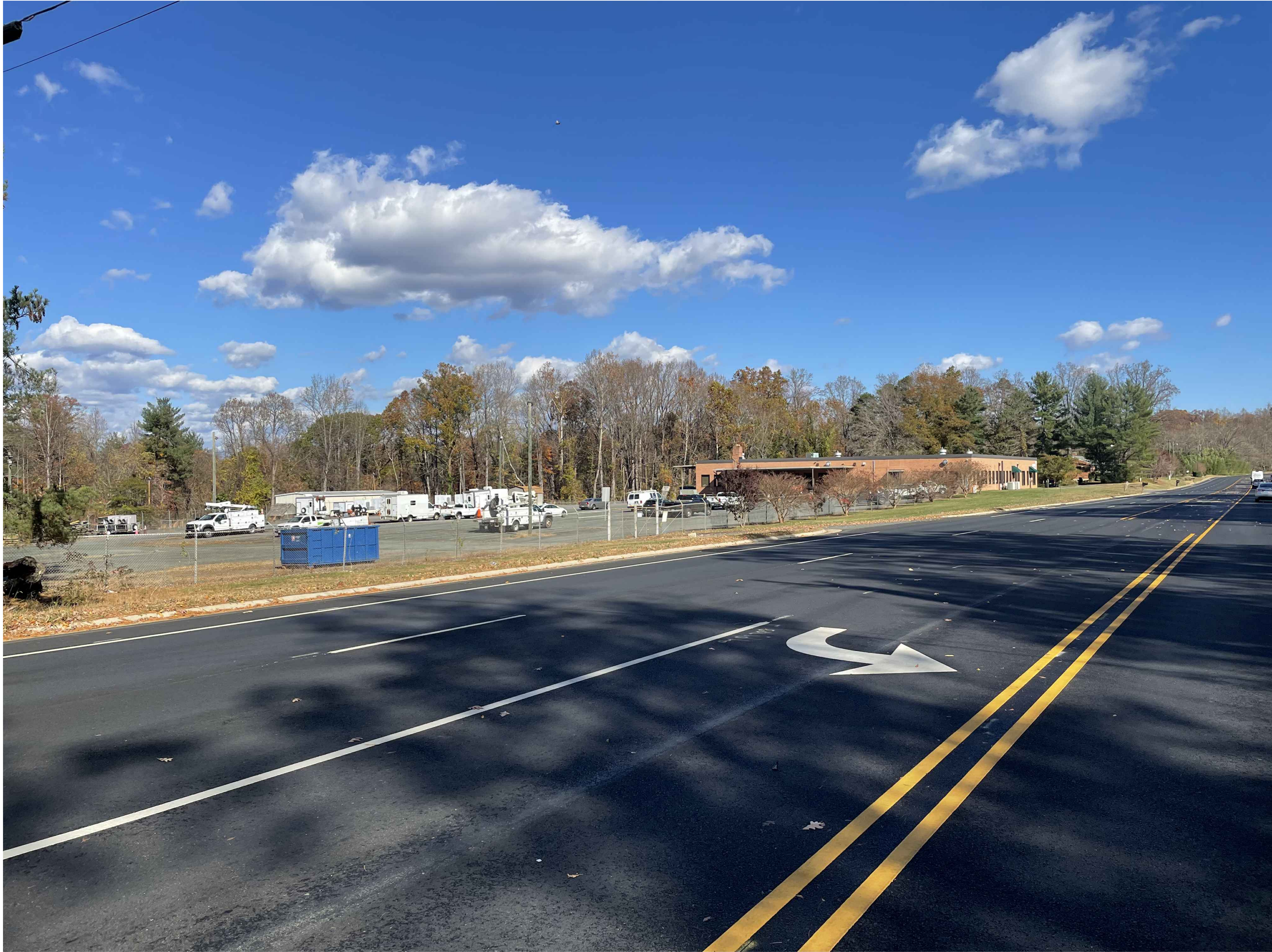
EXISTING FRONTAGE CONDITION - WEST ENTRANCE VIEW
