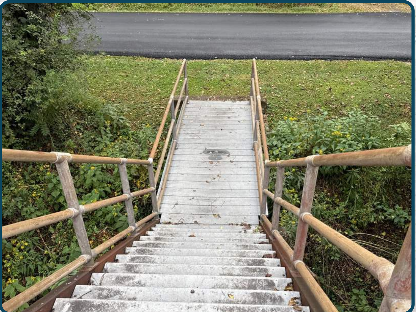
Existing Stairs and Pedestrian Bridge Over Railroad
