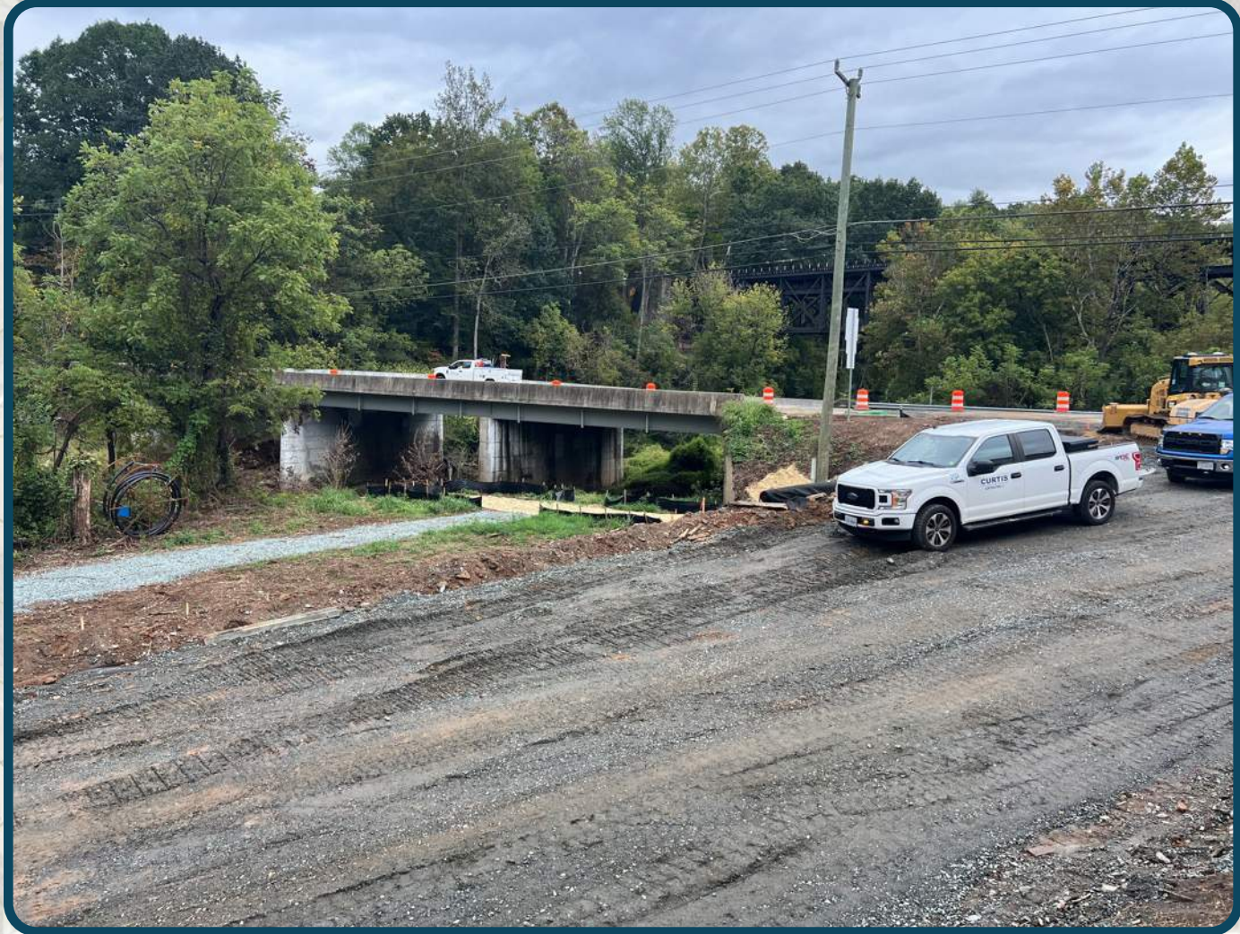
Construction on Rt. 250 - Rt. 240 Interchange
