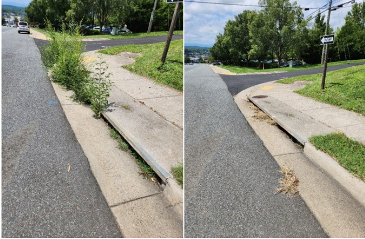
Pantops storm sewer curb inlet:
