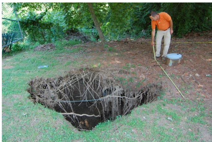
Figure 3: Sinkhole caused by failing underground infrastructure.
