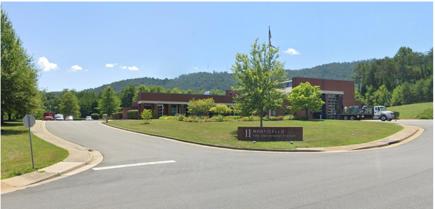
Image: Albemarle County Monticello Fire and Rescue Station
