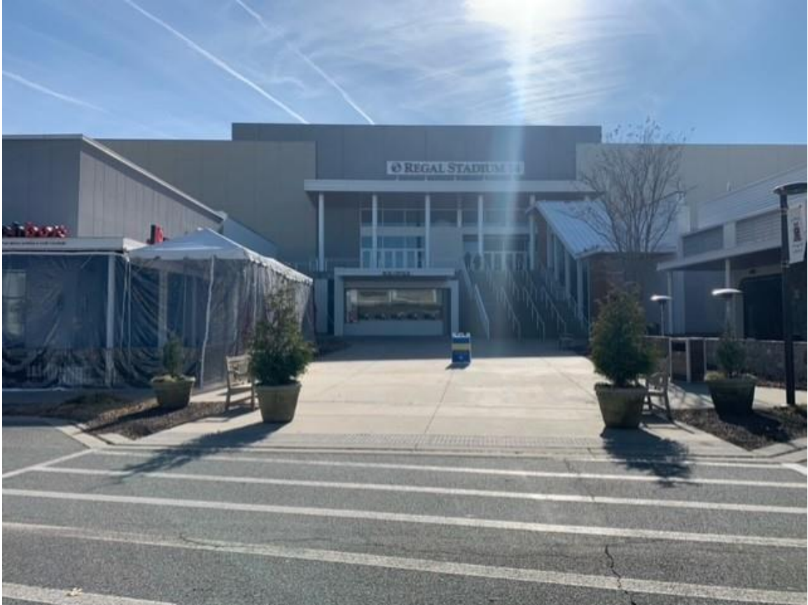
Entrance to parking garage under movie theater.
