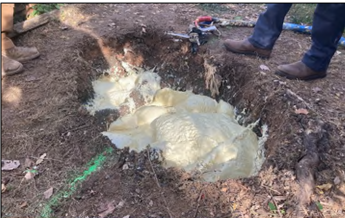
Polyurethane Grout Injected into Sinkhole
