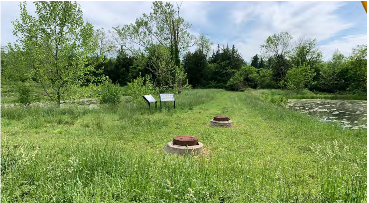
County-owned stormwater wetlands off of Crozet Avenue
