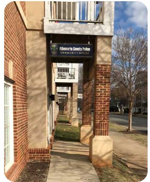
ACPD Community Office in Old Trail
