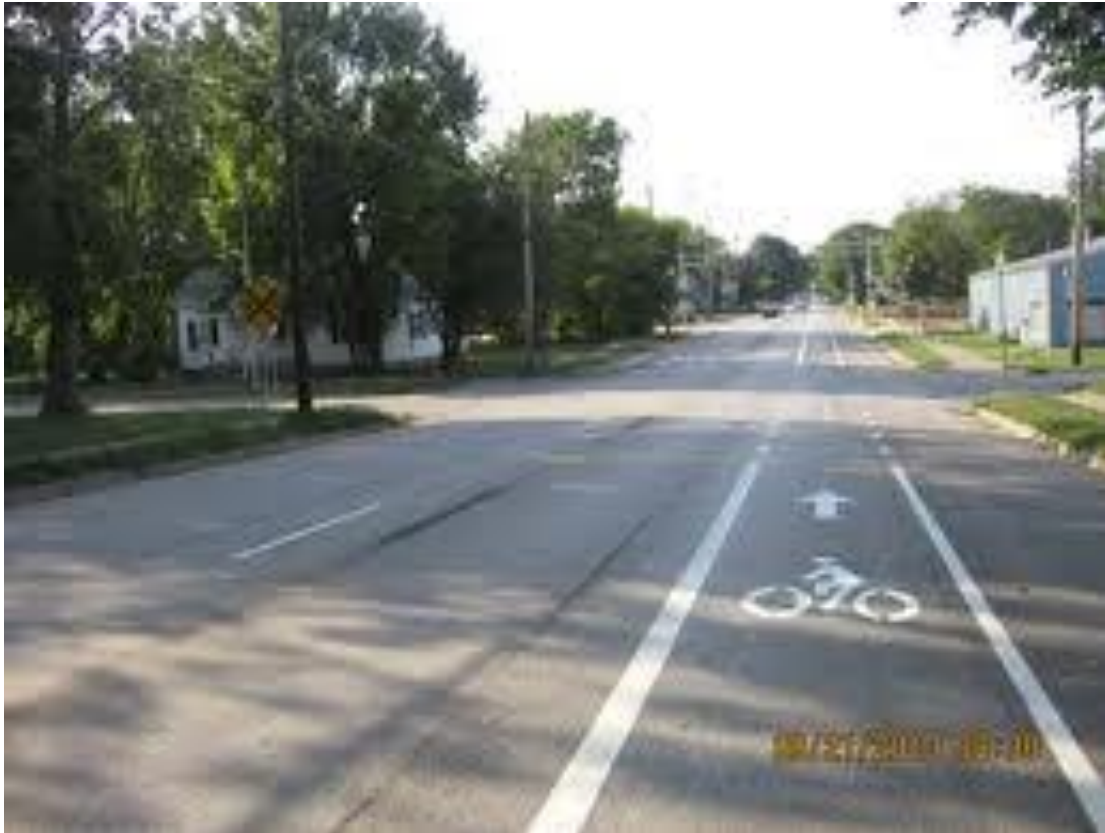
Figure 2.4 – Narrow travelway by re-stripping pavement for a bike lane
