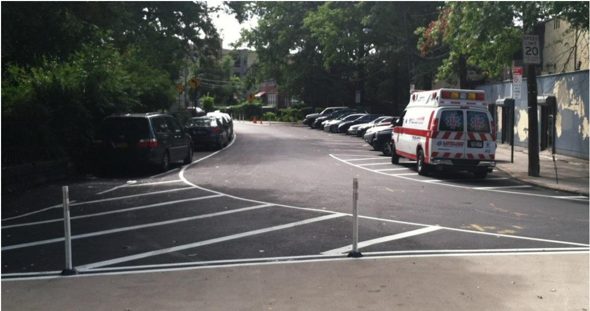
Figure 2.2 –Narrow travelway by re-striping pavement
