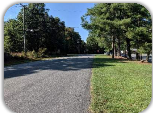
Photograph 4: Southbound Approach – Earlysville Forest Drive
