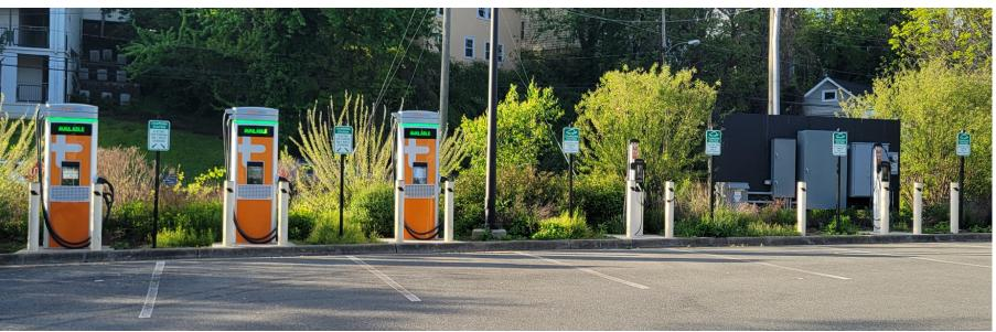
Level 2 Charger – Adds about 39 miles of range per hour. It uses either a commercial EV level 2 charging station or a 240V outlet. These are the most common type of chargers.
