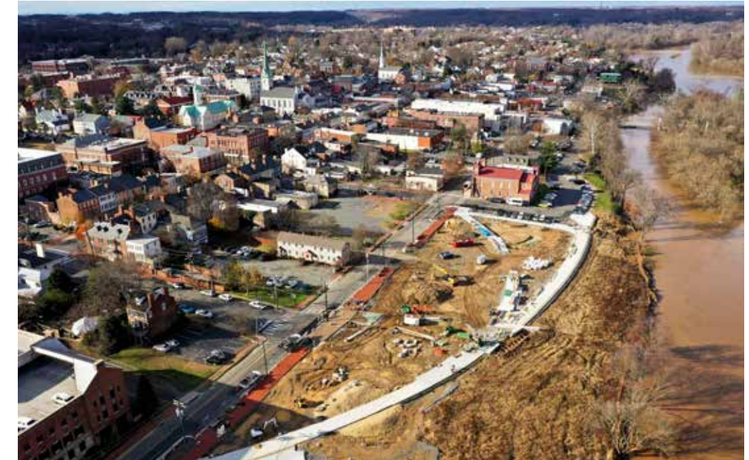
Construction of Riverfront Park in Fredericksburg: Image courtesy of fredericksburg.com
