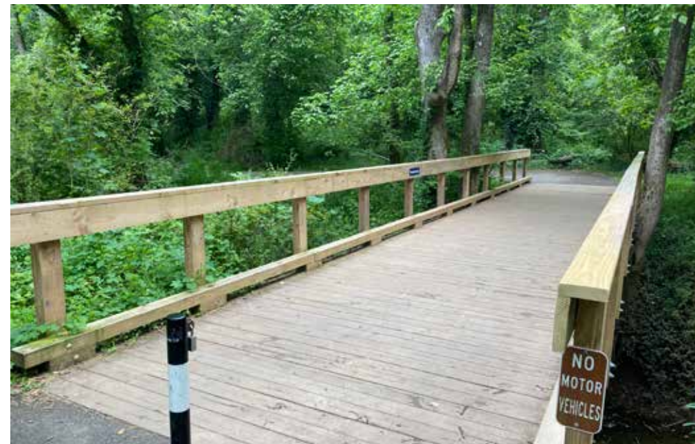
Bridge along Rivanna Trail
