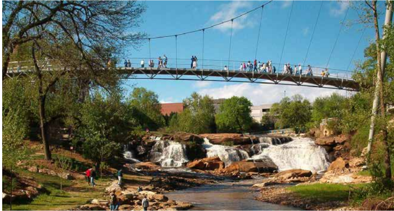
Liberty Bridge: Image courtesy of structurae.net
