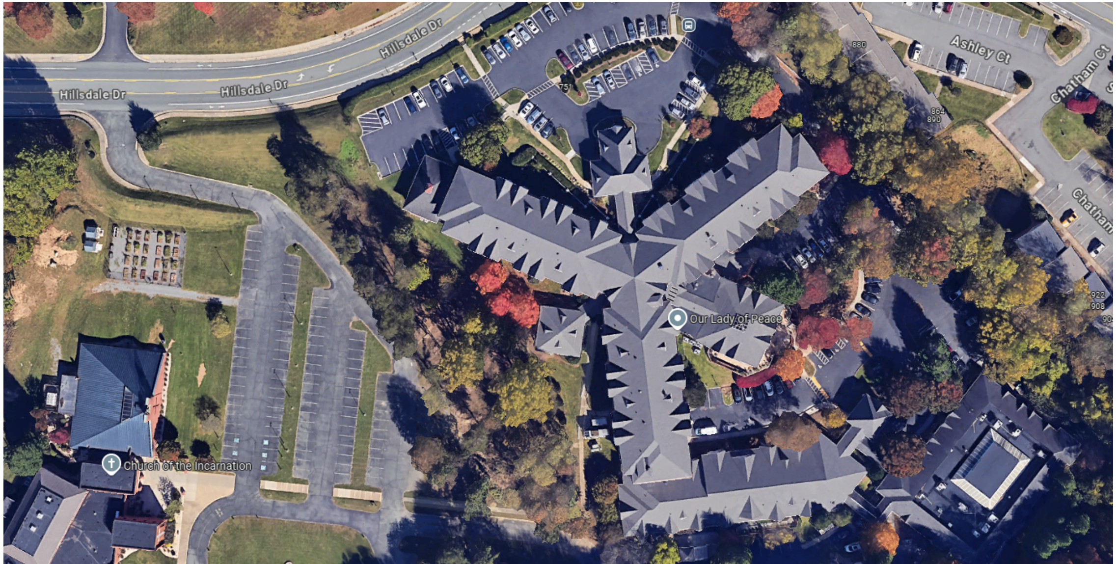
Existing Building in Relation to Church Property
