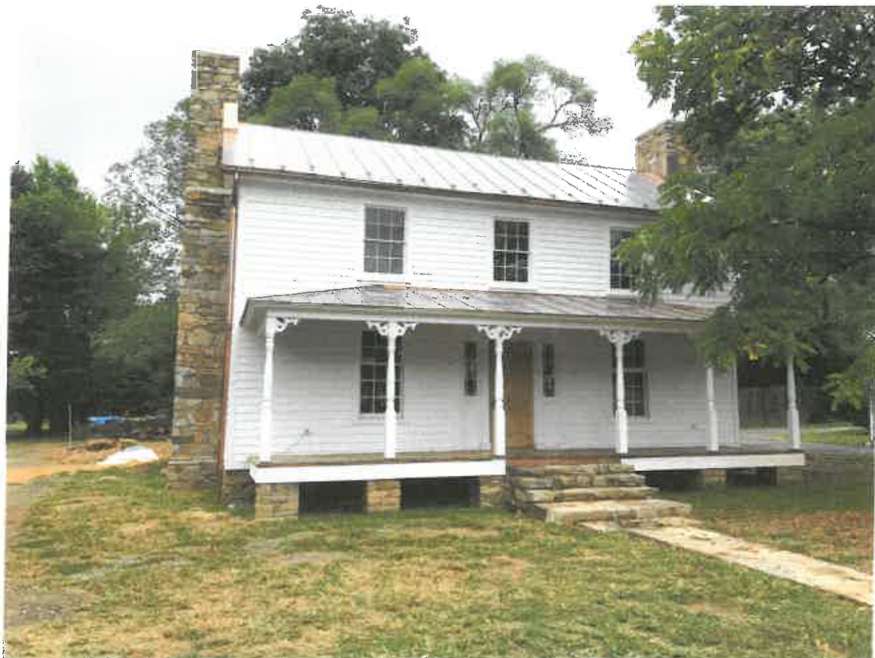
Figure 3: Restored House at 1278 Crozet Ave (front)
