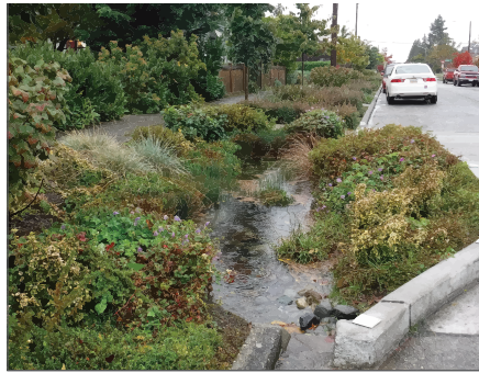
Stormwater Control Measures
