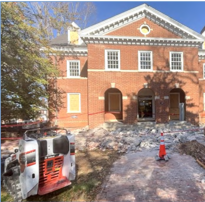
Exterior Concrete Demolition
