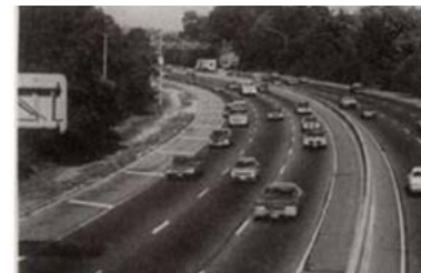
Level of Service B: Stable traffic flow with a high degree of freedom to select speed and operating conditions but with
