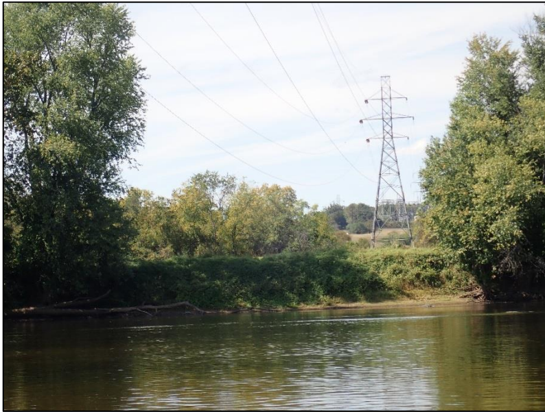
Image 27. Large powerline between Warren and Scottsville.
