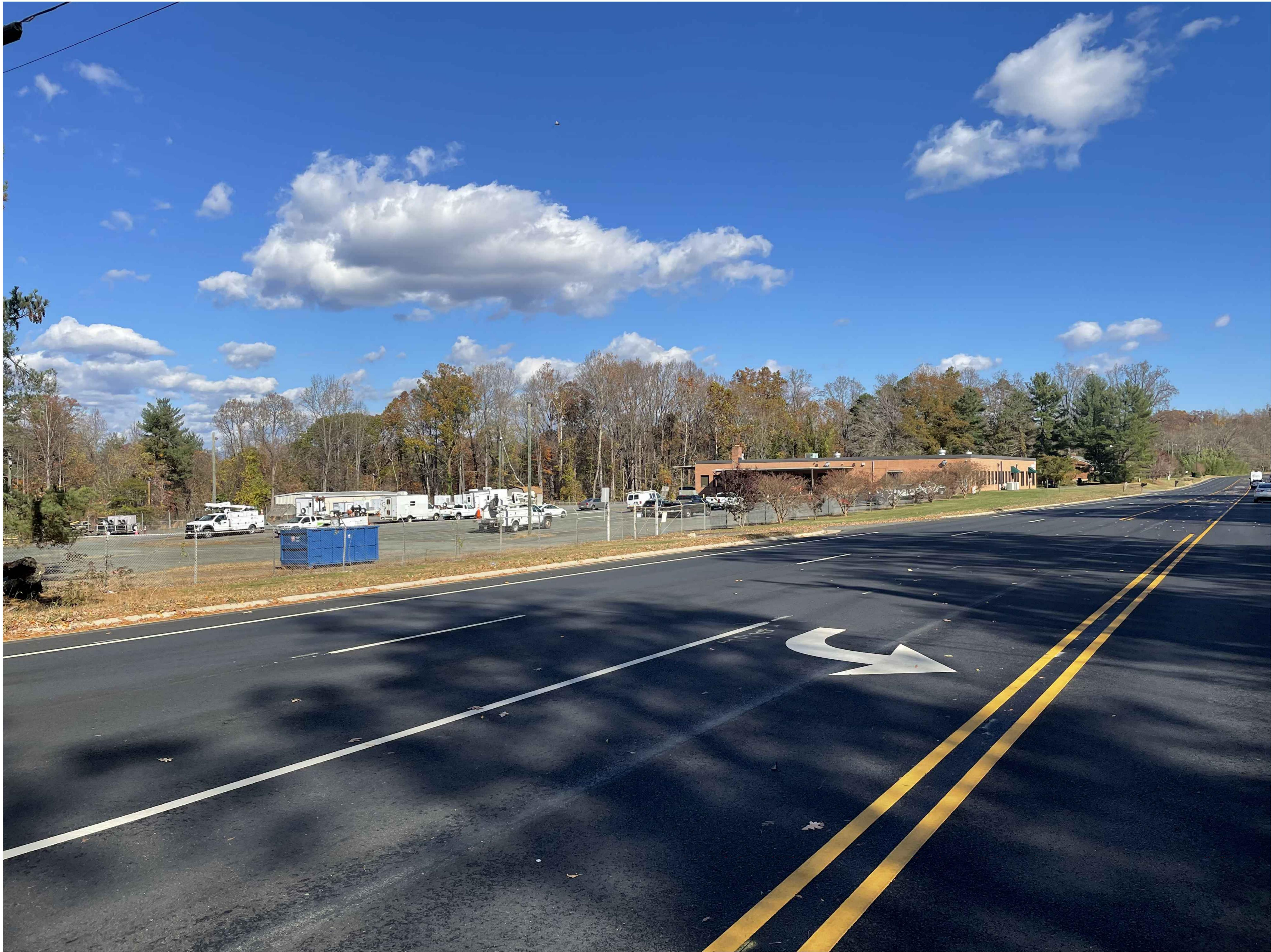
EXISTING FRONTAGE CONDITION - WEST ENTRANCE VIEW
