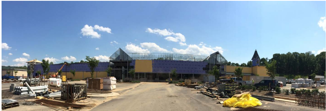
Albemarle County Wegmans under construction
