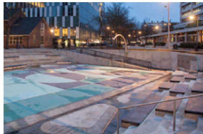
Water Square Benthemplein Floodable Park
