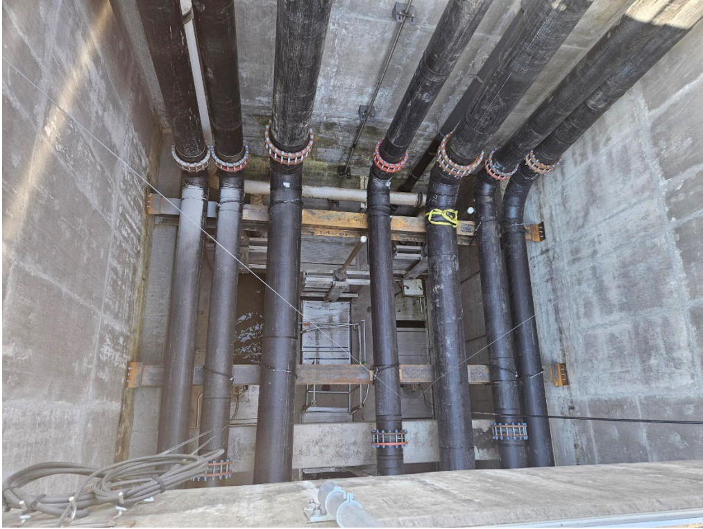
Bypass system pipes in the wet well.
