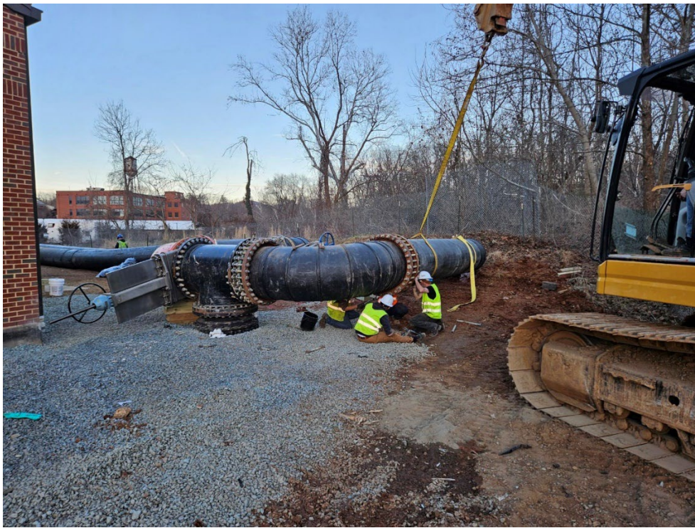
Bypass system pipes.
