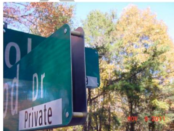
Figure III-8 Oversize Sign Showing Corner Attachment Detail
