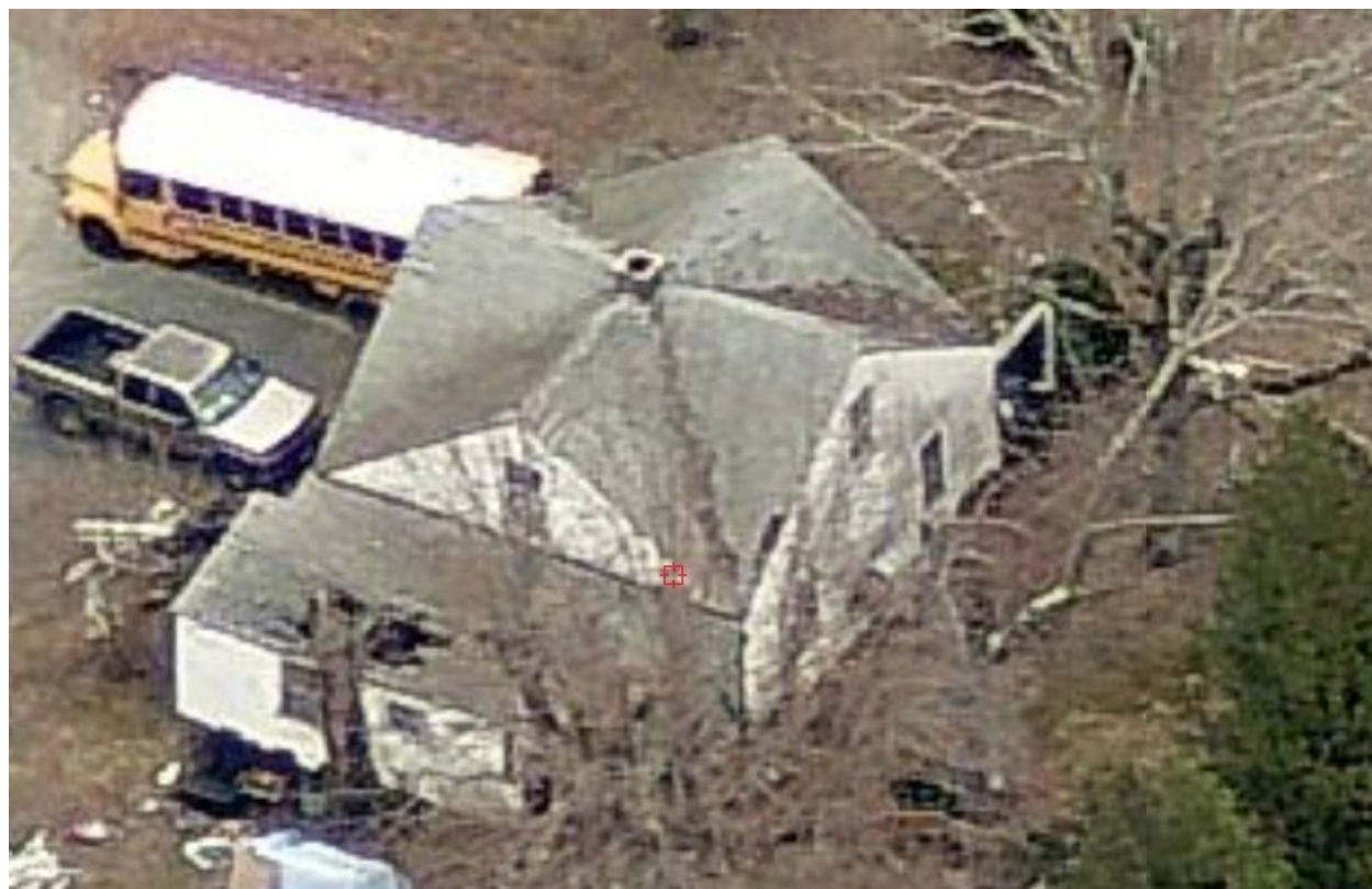
Att. B – Property conditions – 8038 Blenheim Rd.
