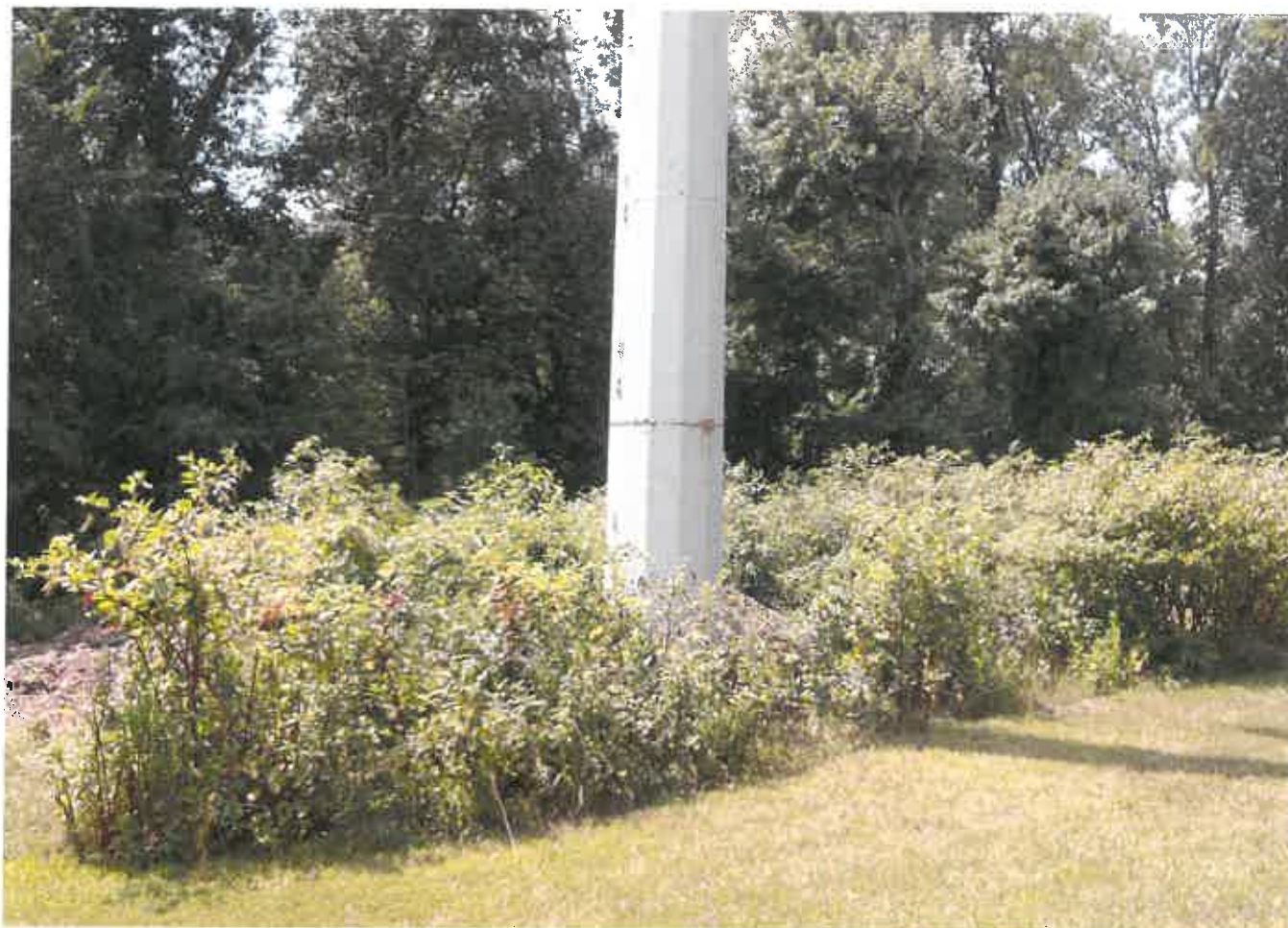
View of the power tower's base and surrounding vegetation within the Dominion Power easement
